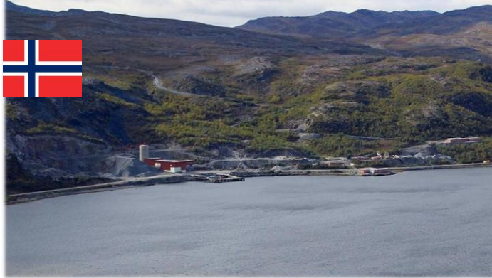
NSG – Underground Exploration -UNDERGROUND TUNNEL PERMITS-
