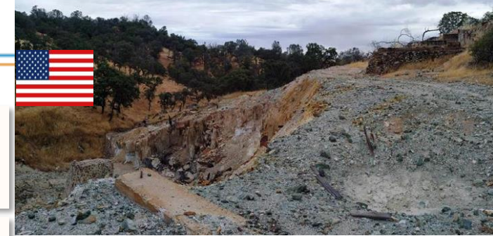
Blue Moon – Ramp In Construction -EXPLORATION RAMP PERMITTED-
